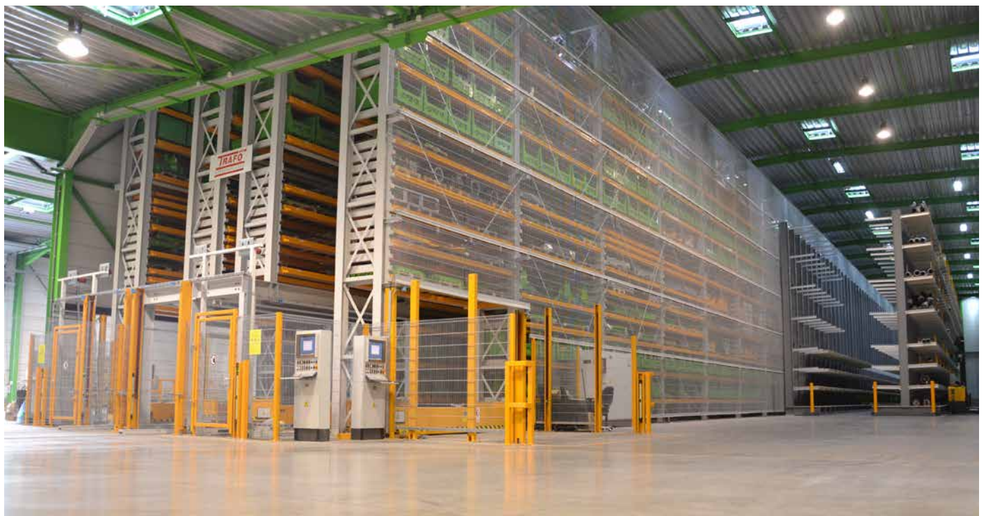
Automated Storage Area of 28.000m 3
